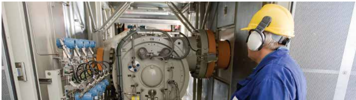
FGSZ staff member controlling the turbine of the compressor at the Hungarian-Croatian Interconnector Gas Pipeline compressor station.
