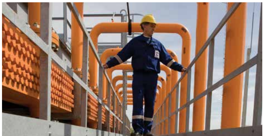
FGSZ staff member checking the cooling system
